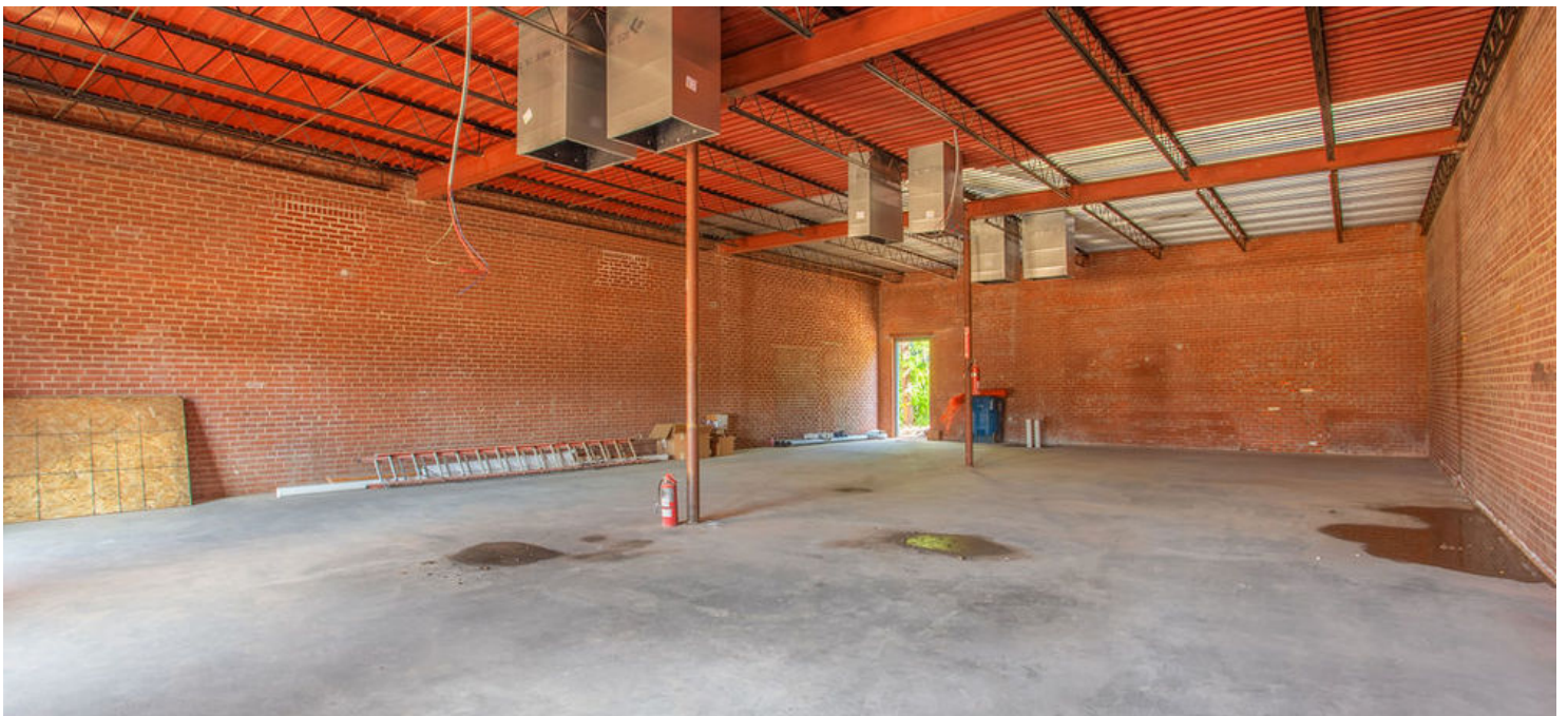
Suite B Interior, under construction
