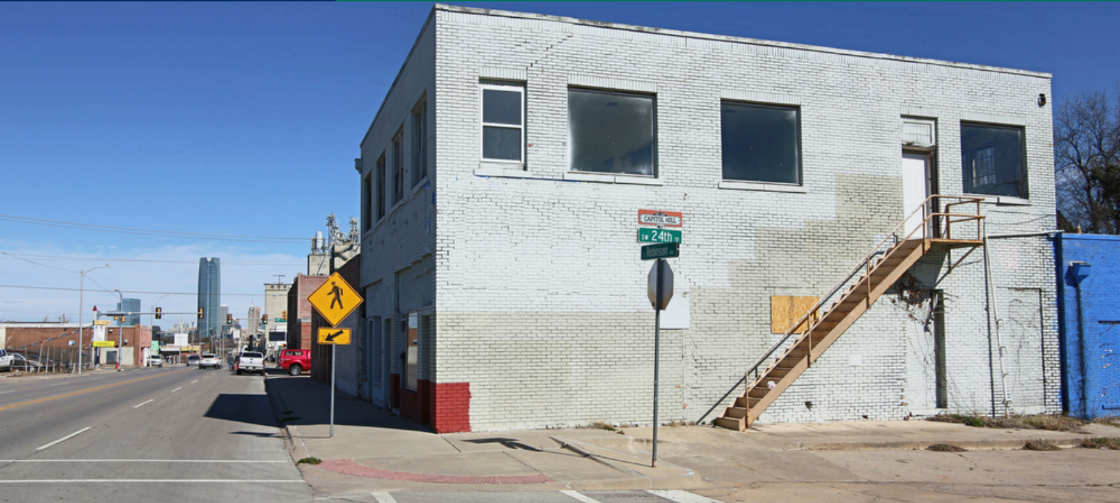
Located at the N/E corner of Robinson Ave & SW 24th
