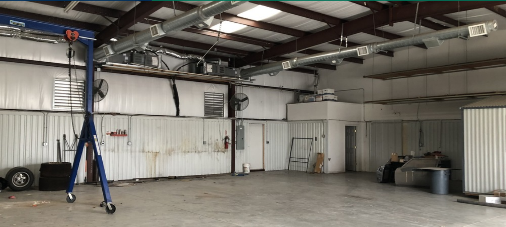
2814 W Reno, OKC | Industrial space for lease - interior photo
